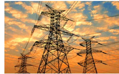
Power Line Inspection
